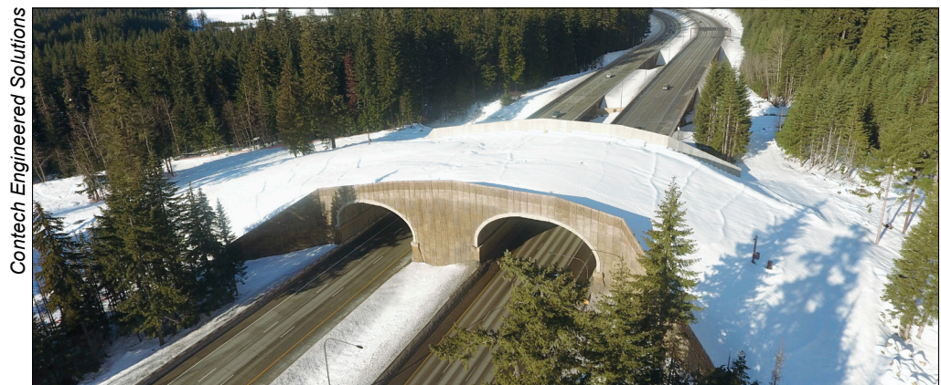
Figure 5—Typical buried wildlife overpass crossing in Europe.
