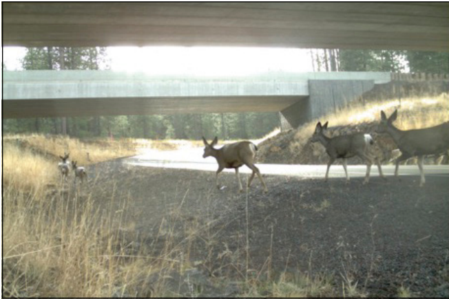
Figure 9—Mule deer walk through an underpass with an access road to Lava Lands Visitor Center on the Deschutes National Forest in Oregon. The twin underpasses under busy U.S. 97 serve animals at night and in the off seasons when the visitor center is closed.
