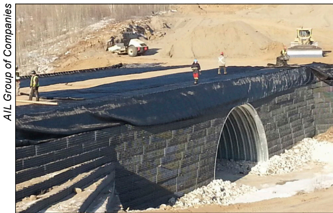
Figure 12—Geosynthetic reinforced soil is used for a buried bridge during construction.
