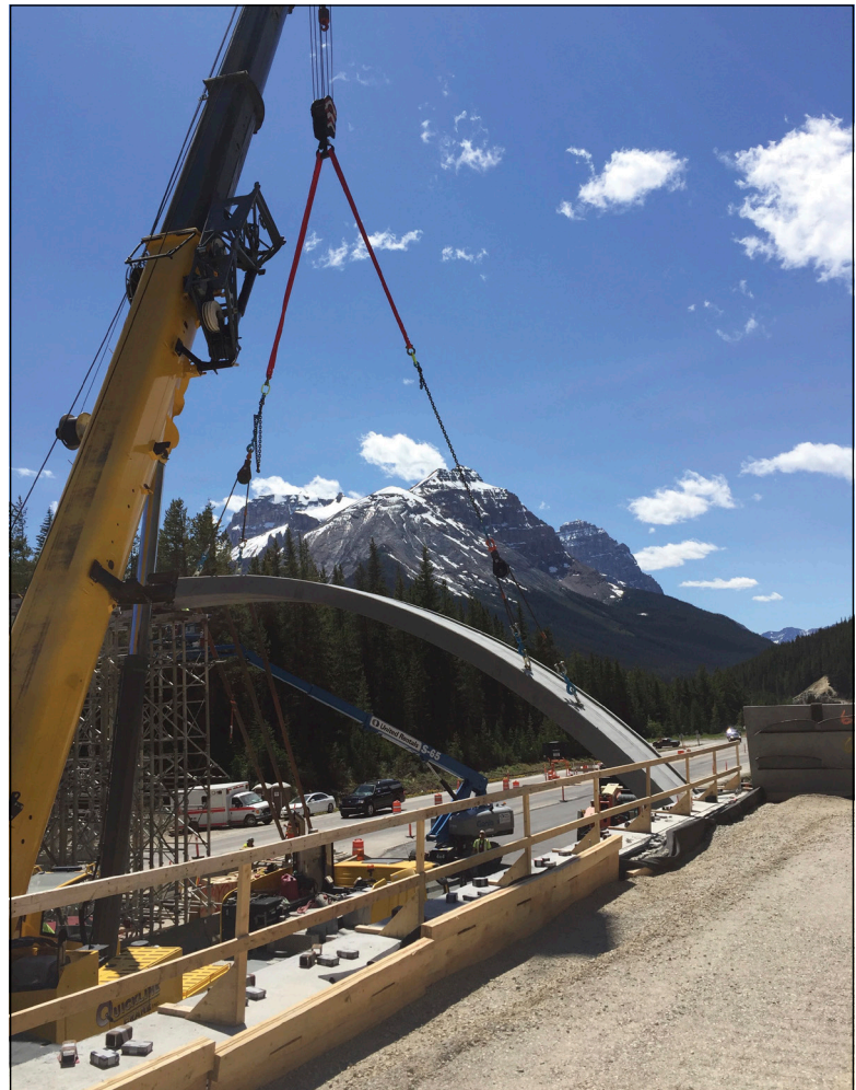
Figure 14—Cranes erecting concrete arches at Trapper’s Point on U.S. Hwy 191 near Pinedale, Wyoming.
