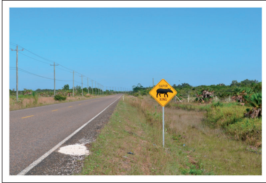
Figure 2. Two sets of reflective wildlife crossing signs were installed at two hot spots identified for tapir-vehicle collisions.
