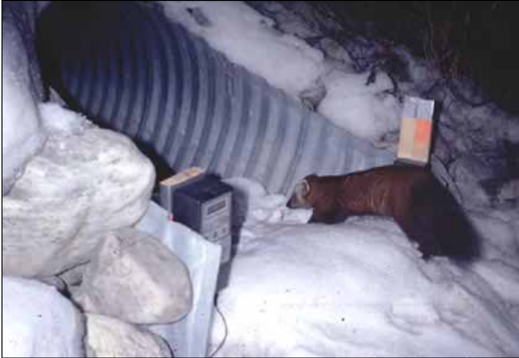
Figure 51. Photo. American marten using a drainage culvert to cross the Trans-Canada Highway, Banff National Park, Alberta (Credit: Tony Clevenger).
