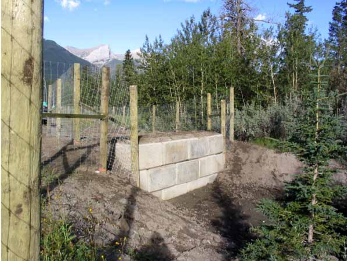
Figure 71. Photo. Escape ramp (jump-out) for wildlife trapped inside highway right-of-way (Credit: Tony Clevenger).
