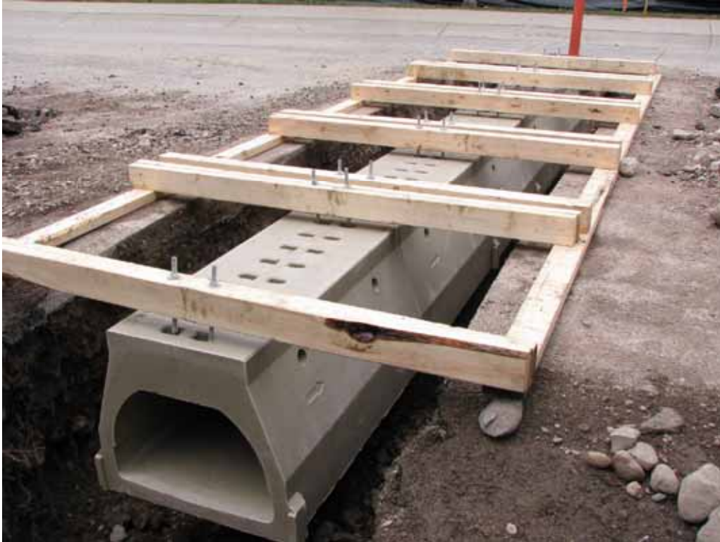
Figure 55. Photo. Construction and placement of amphibian tunnel in Waterton National Park, Alberta (Credit: Parks Canada).
