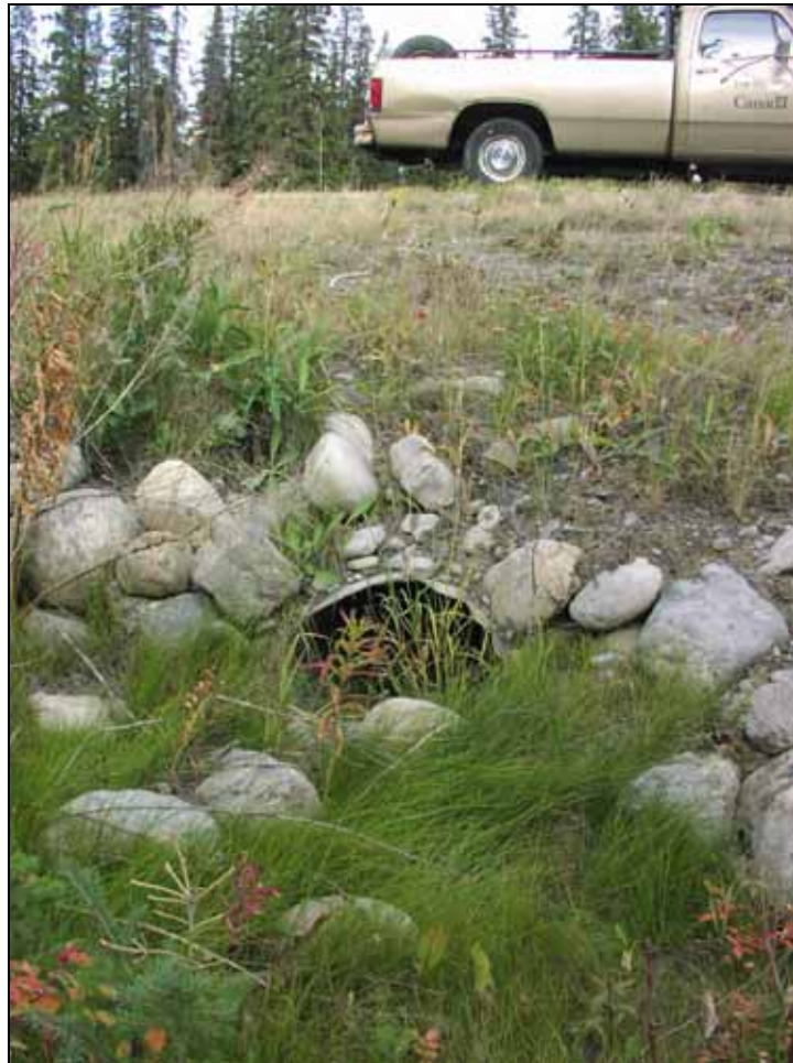
Figure 49. Photo. Small- to medium-sized mammal underpass (Credit: Tony Clevenger).
