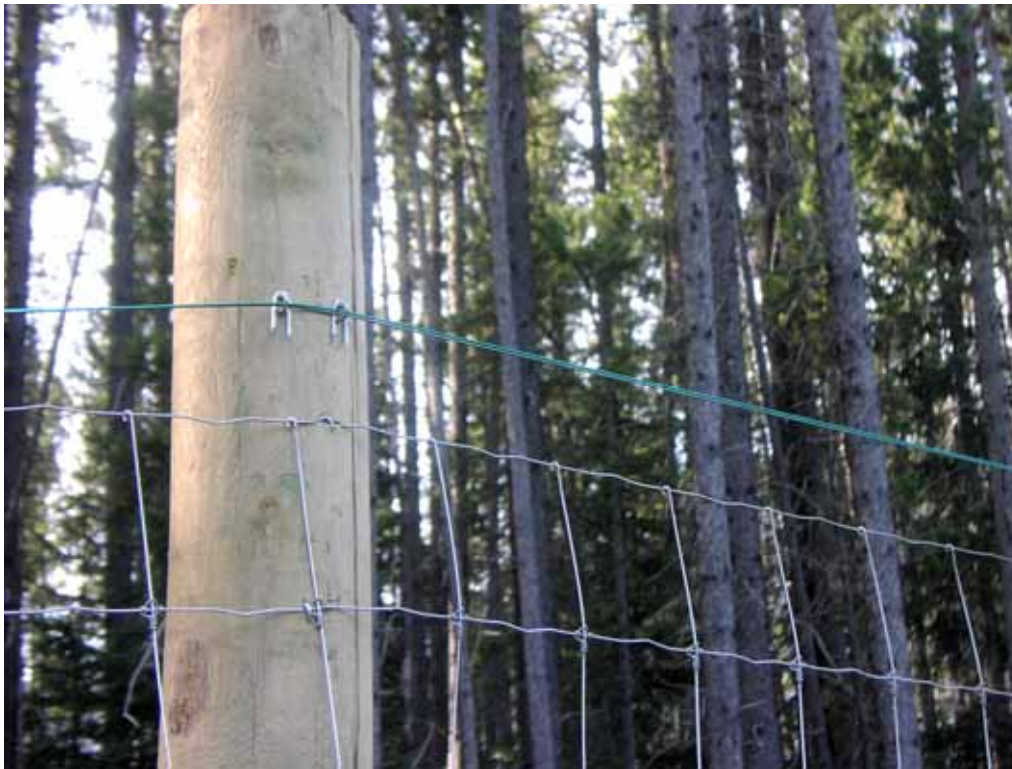
Figure 67. Photo. High tensile cable designed to break fall of trees onto fence material (Credit: Tony Clevenger).
