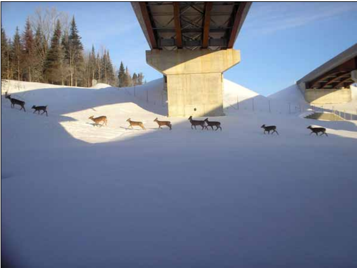
Figure 39. Photo. Viaduct as wildlife underpass (Credit: Ministère des Transports du Québec).
