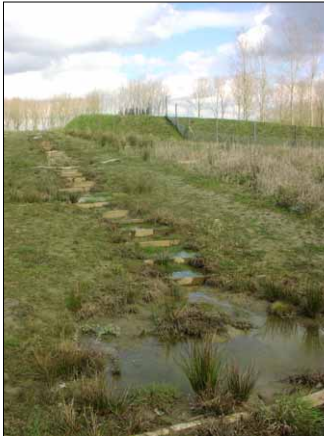
Figure 42. Photo. "Stepping stone" ponds on wildlife overpass used to assist amphibian movement (Credit: Tony Clevenger).
