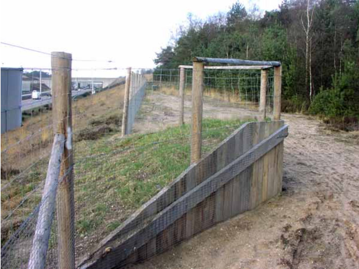
Figure 73. Photo. Wildlife escape ramp (jump-out; Credit: Tony Clevenger).
