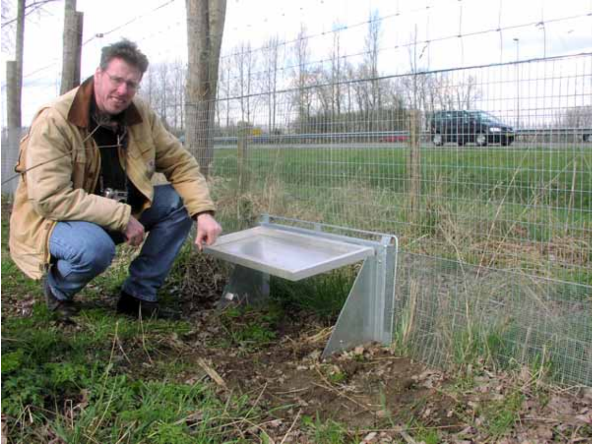
Figure 74. Photo. Hinged door for escape of medium-sized mammals (Credit: Tony Clevenger).
