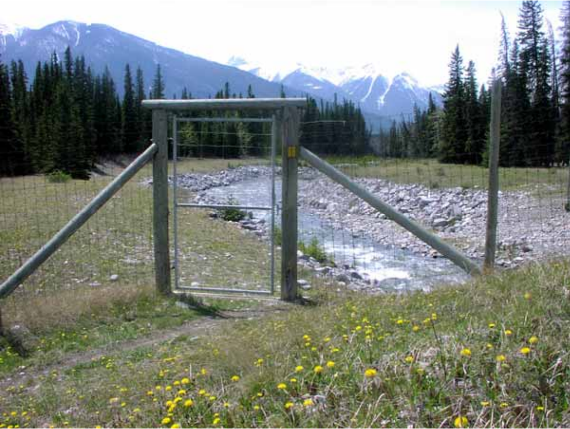
Figure 72. Photo. Single swing gate in wildlife exclusion fence (Credit: Tony Clevenger).
