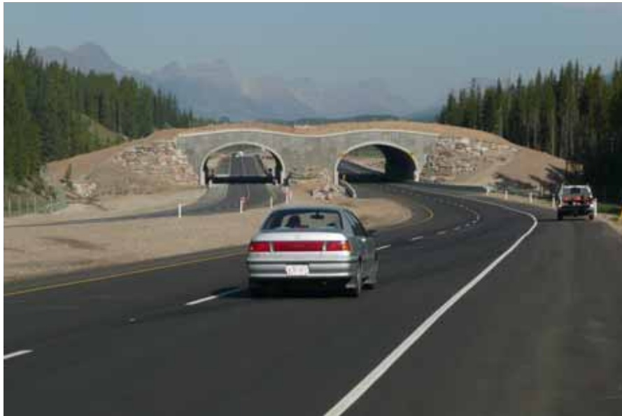
Figure 33. Photo. Recently completed but unlandscaped wildlife overpass (Credit: Tony Clevenger)
